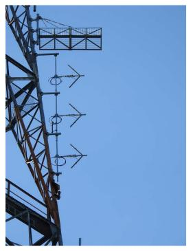
The Ice shield should be installed above the antenna as per the spacing calculated to ensure minimal interference with your antenna system.
