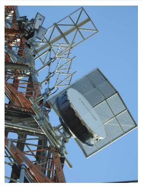
The Ice shield will extend past your antenna system to ensure any falling ice cannot come into contact with your system.
